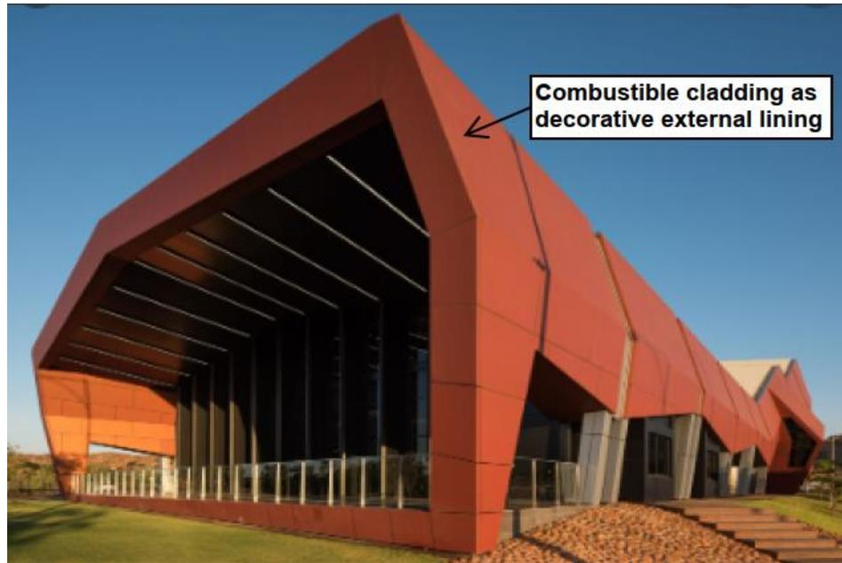
**Figure 2 – Photo showing external combustible façade of a building used as a weatherproof and decorative lining**
